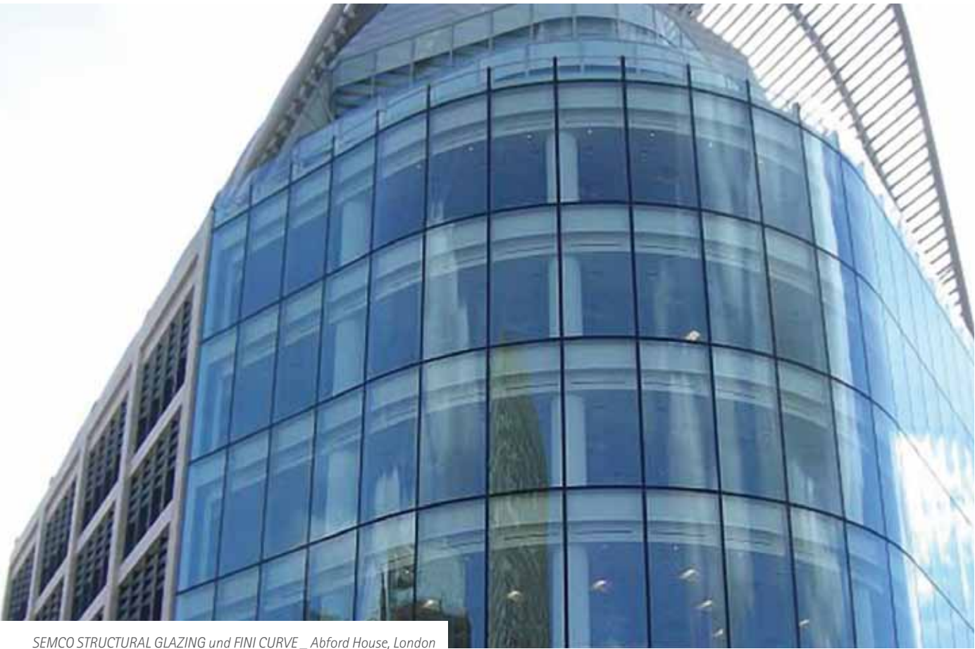
SEMCO STRUCTURAL GLAZING und FINI CURVE _ Abford House, London
